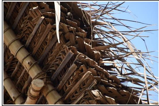
A piece of ground, 5 by 7 meters was prepared and stone pillars erected as plinths along the sides and inside. Long relatively thin pine members were then placed on the pillars to form the base for the upper floor and the roof. Everything was tied together with ropes made of coconut fibres. The roof finally was covered by dried coconut leaves. All very simple.
