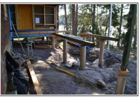
Two of the old concrete plinths needed to be lengthened and I also needed to cast two completely new ones.
