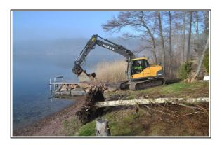
To make space for the new house section we took help of a 14 ton Volvo excavator. He uncovered the ground so I could cast the plinths needed as foundation for the new building.
