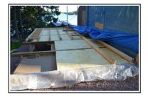
With the old house section gone I hired an 8 ton excavator to remove the soil and prepare the foundation of the new building. We soon found solid rock, which is nice to build on. The old house stands on plinths and I could reuse some of them but had to add 6 new ones. After that I started the construction of the new floor with 35 centimetres of heat insulation.
