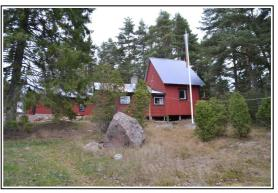
Summer passed quickly and it was soon time to finish the exterior of the new house before the cold season. I purchased 950 meters of 22X120 mm wooden panel from a local lumber mill and Tove painted, first with oil and then with traditional red. A few thousand nails later the outside of the house was ready to meet the winter.
