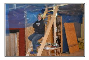
With the exterior finished I moved inside and continued working. Heat insulation, plastic film, inner ceiling, a temporary stairway to the attic and so on. Tove seems happy with the result.
