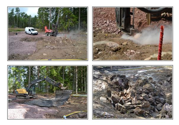
In order to get the new house down to the right ground level we had to call a rock blaster. He drilled around 40 holes, loaded with dynamite and covered them with rubber mats before he pressed the button. The result was perfect.
