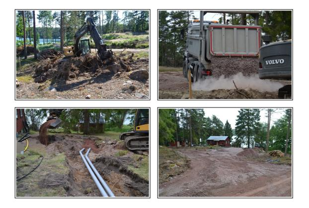
I was lucky to get in contact with a very experienced excavator driver. He had a 14 ton Volvo crawler and did all the digging for us. First he removed all the pine stumps and roots, then he prepared the new entrance from the road and covered with gravel. He also made a ditch to the old house so that we could connect the new waist system, water feed and electricity.
