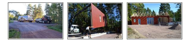
The house was delivered as a kit of seven wall sections, prefab rafters, doors and a lot of other stuff. 8 hours after the truck arrived, the house was mounted with all rafters in position.
