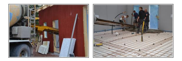
Floors were isolated with 100 mm of styrofoam, reinforced with steel grating and covered with 100 mm concrete. It took 4 men one day to complete this.
