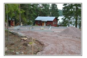
We hired a local building construction company to help us with the house. First step was to make the foundation. Concrete plus two layers of Leca blocks.
