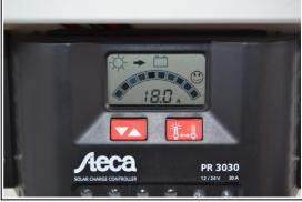
Another job was the fitting of a new 100 watt solar panel. We now have 6 panels with a total rating of 360 Watts. A new larger regulator was fitted to cope with the increased power.
