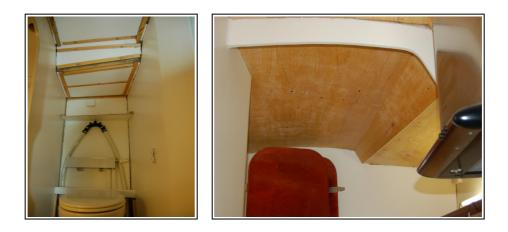
Another job that has now started is finishing the inside ceilings. There is 20 millimeters of heat insulation on the inside of the deck everywhere and to cover that there is sheets of 6 millimeter plywood treated with epoxy to be waterproof.
