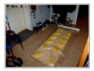
Mould (mögel) can be a problem, specially under a bed. The solution is ventilation. Therefore all beds in Bird of Passage have double bottoms with air ventilation. On this picture you can see how I glue the two pieces of plywood together with thin strips between. Lead weights and a plane floor keeps everything in position. This is the lower bed of the center cabin, named Gustav's cabin, our youngest son.
