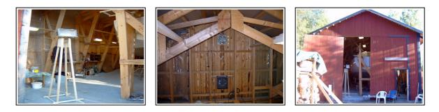
Good light is important. I used a 1500 watt halogen lamp ! That helped a lot. Good ventilation is also important. I installed two fans in one of the gable walls of the boat house and opened the other gable. The result was a steady stream of air along the length of the boat that very effectively removed all vapors in short time. A breathing mask with coal filter is also needed of course.
