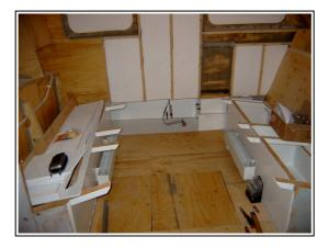
Here is a final picture from the deck house showing two convectors mounted and connected and also the defroster unit though not yet connected. I'm close to have finished the heating system !!!!
