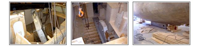
The keelbox weighs approx. 1300 kg, is 3 meters long and 2.3 meters high and there is not much room inside the boat so it took some time and maneuvering until the keelbox was in a position where it is standing on the floor of the boathouse. Next step is lifting the boat 1 meter up in the air so the keelbox will rest on the wooden floors inside the boat. This is how it looks from the outside after lifting the boat half way up.
