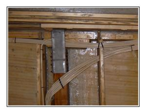
Before putting the plywood pieces back for good I have to finish everything else that fits behind them. One such thing is the tubing for the electrical system where I used 16 millineter PVC tubes of the same kind used for electrical systems in homes or industry. There will be a 12 Volt DC system and a 230 Volt AC system. There are also tubes for different instruments or gauges and I also add an extra tube here and there for future use.
