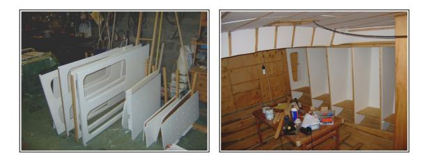
After having finished most of the electric tubing I now work with the inner walls closest to the hull sides. These are made from 12 mm plywood, coated with one layer of epoxy, painted white and with foam glued to their back sides for heat insulation and flotation. To the right is a view of the aft cabin right now. Note that there is also heat insulation mounted in the ceiling, 20mm. So far I have approx. 1.5 m3 flotation in place.
