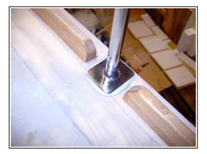
Another thing that has to be finished before putting the plywood back is to finally fasten all deck gear that is screwed through the deck/sheerclamp. One
