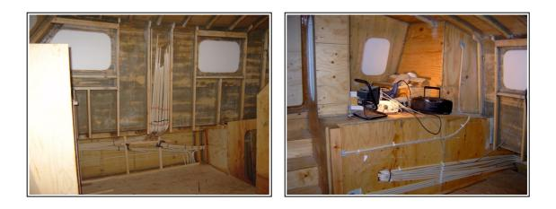
Most of the pvc tubes for the electric system are now in place, almost 300 meters ! Many of them go to the main control panel close to the indoor steering position. Others go to the 2 main electric central junction boxes in the machine room. Some of the tubes are for the 230V AC system and some of them are for the 12V DC system.
