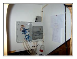
A basic 230V system is now running. This means I can now connect lamps and tools to the boat system and don't need long cables hanging everywhere. This makes life a little easier working inside the boat. It also makes life safer since there is plenty of fuses and also the RCCB.
