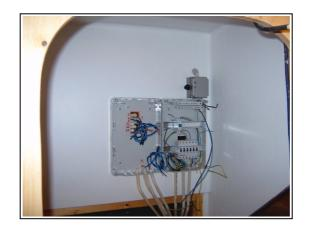
There are two junction boxes in the machine room, the one to the right in the picture is for 230V AC and the other one is for the 12V DC system. The 230V box includes a number of automatic fuses, a 30 mA Residual Current Circuit Breaker (RCCB) and a control lamp that shows when current is available. 230V AC will either come through the shore line or from a 12V
