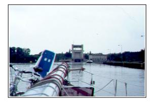
Here comes a more normal lock but still very large. The lock gate opens upwards so you go under the gate into the chamber.
