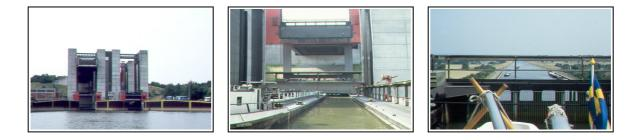
Lubeck-Elbe Canal connects Lubeck with the River Elbe. A short distance downstream of Elbe, the Elbe-Seiten canal begins which is large and wide and relatively newly built. No lock is the other alike. Here is an unusual kind of lock that acts as a lift. You go into a huge "bathtub" which is then lifted 38 meters up in the air by 4 huge chains. There are two similar elevators next to each other. One goes up when the other goes down.
