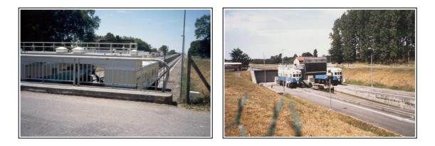
There were many locks and most of them were of pretty ordinary design but this one was something extra. Based on the principle of a ramp with vertical sides, two heavy tractors, one on each side of the groove, carry a retractable lock gate between them. A boat comes in, the gate is lowered behind the boat and the tractors start pulling the water and the boat upwards.
